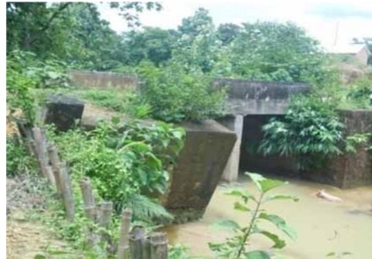
**Non rectifiable damaged CD**
