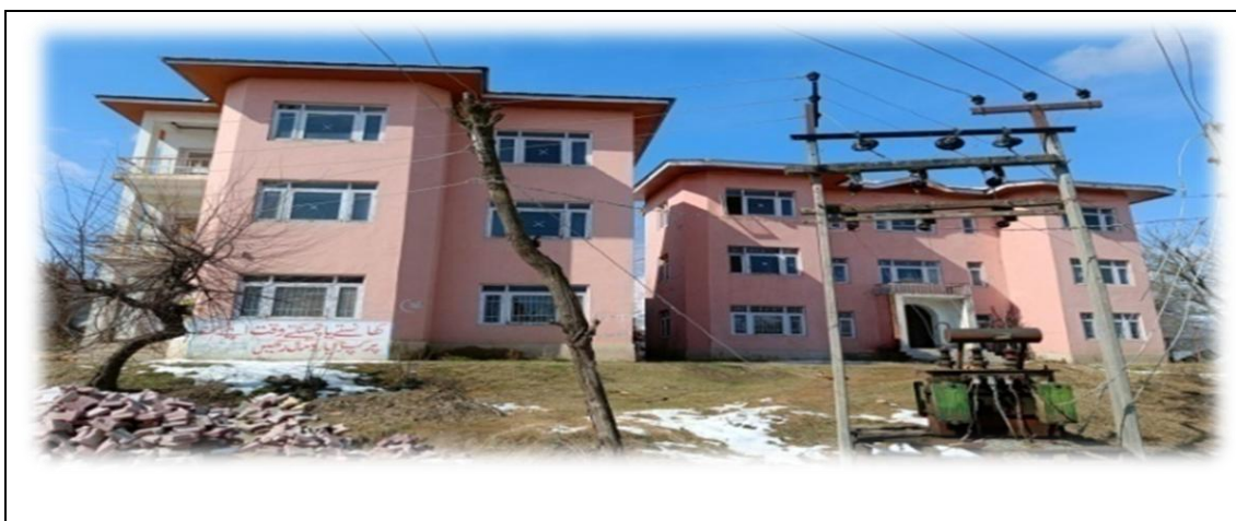
Vacant staff quarters at PHC B. Kalan
