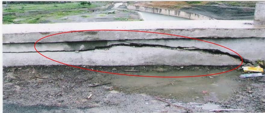
**Crack developed in the retaining wall**
