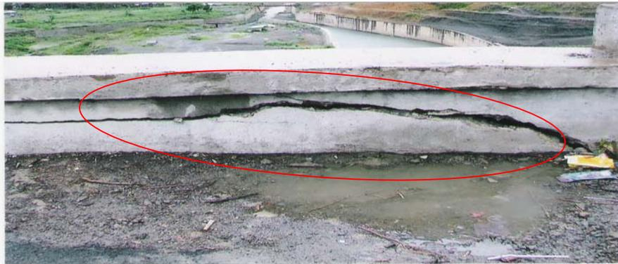
**Crack developed in the retaining wall**
