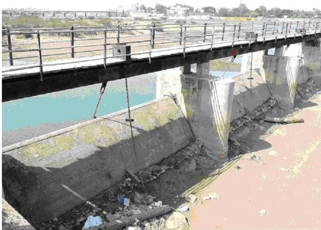
(Photograph showing non-functioning of Gates due to trash/bushes getting stuck in the axle)
