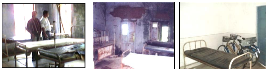
(Inside view of dilapidated wards of PHC, Barharwa (Sahebganj), PHC, Bharno (Gumla) and APHC, Kenduadih (Dhanbad) L to R)
