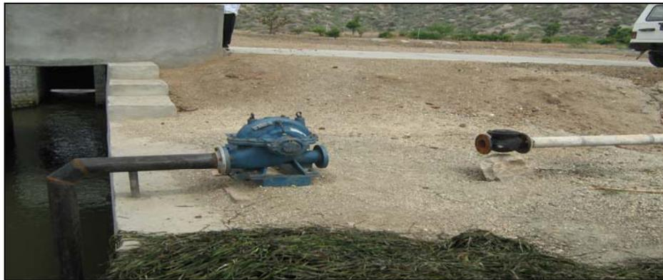
Photograph showing non-connection of rising main of water supply scheme with source (06.07.2010)
