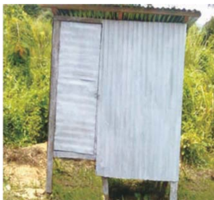
Separate Girls Toilet at Chamdurtlang Primary School constructed on the instruction of Executive Member (i/c Agriculture) LADC, Lawngtlai during 2010-11
