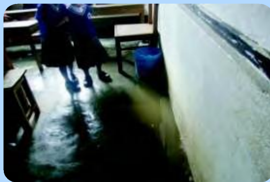
Rain water leakage in the class of Panthang PS, East
