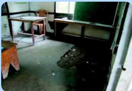
Damaged flooring due to leakage of rainwater in Yalli PS, East
