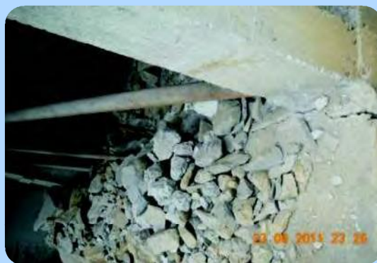
Crack in the RCC structure
