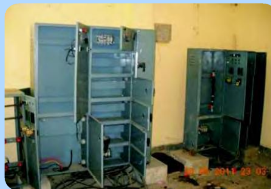
Electrical equipment without components
