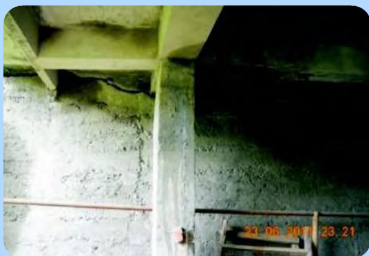
Crack in the RCC structure
