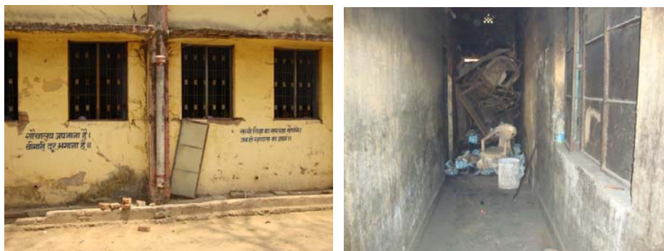
(Photographs taken on 4 May 2011 showing dilapidated building of OBC girls' high school with hostel presently running in the hostel of K.B. Women College, Hazaribag)
