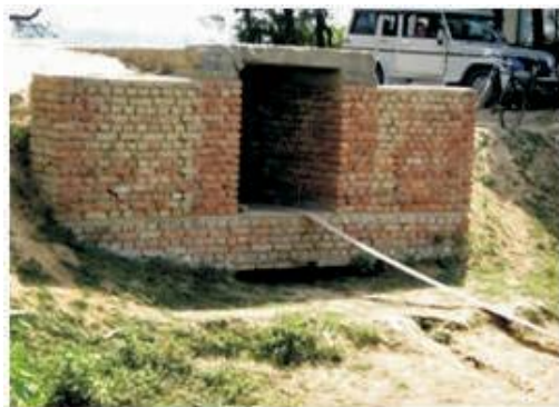
Scheme No.8/10-11 PS-Lakhnaur: Foundation was not constructed
