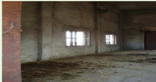
Pump house at Rudur without pumps
