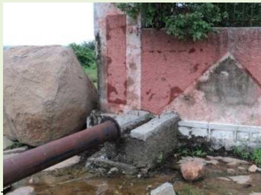
Pipeline from CPWS Vattinagulapally upto boundary wall of Osman Sagar Reservoir awaiting connectivity
