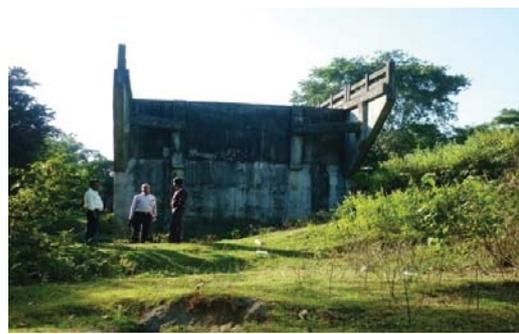
*Incomplete earth work for bridge approach without any retaining wall and protection work on Simaluguri side. (November 2012)*
