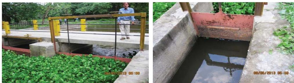
*Fully closed Cross Regulator of the Headwork      Head Regulator at the Headwork
