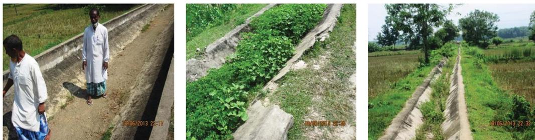
*Damaged and Idle Main as well as Branch Canals under the schemes
