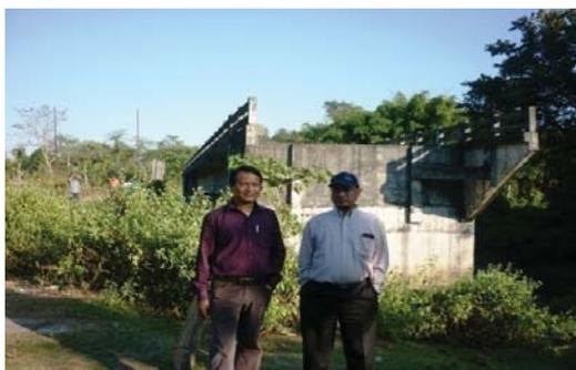
*Bridge proper without any approach and protection work on Sonari side. (November 2012)*
