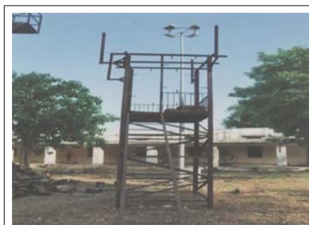
Picture showing broken watch tower at Sabarmati CP (20 May 2013)
