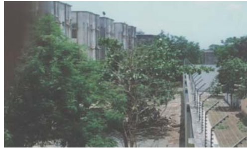
Photograph of police staff quarters constructed near to main wall of Navsari Sub prison (4 May 2013)
