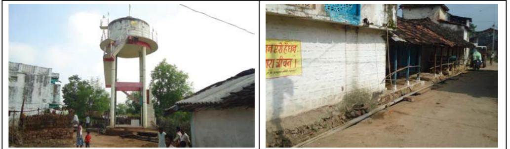
Over Head Tank constructed and GI pipeline can be seen layed at a cost of ₹ 6.50 lakh in October 2011 within village Ratanpur Girdhari, Raisen District from where household connection are provided. The PWSS is handed over to Mendki Panchayat of the village, having 115 individual household connections.
