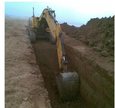
*Excavation of vertical chimney by mechanical means*
