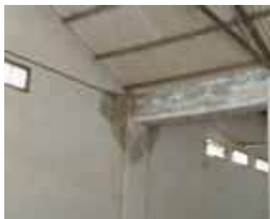
Picture 6: Leaky roof in Namakkal WH
