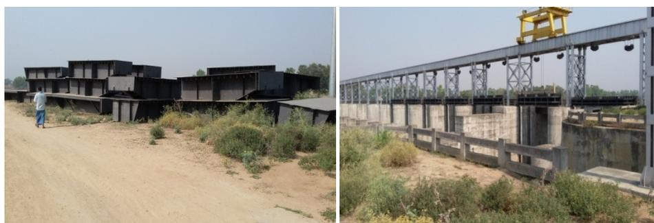
*Photograph of Punpun Barrage showing incomplete erection work of the barrage*
