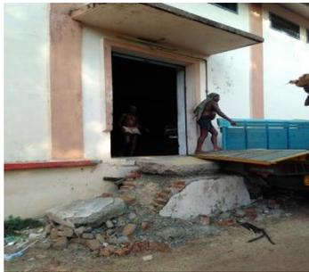
**Picture 8: Damaged platform in Tiruvarur WH**
