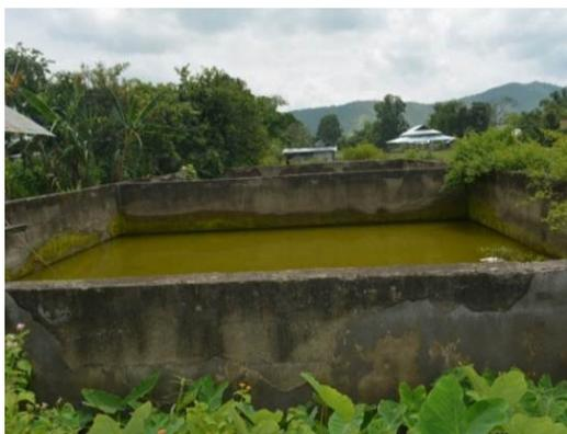
**Deplorable condition of Slow sand filter for treatment of raw water**
