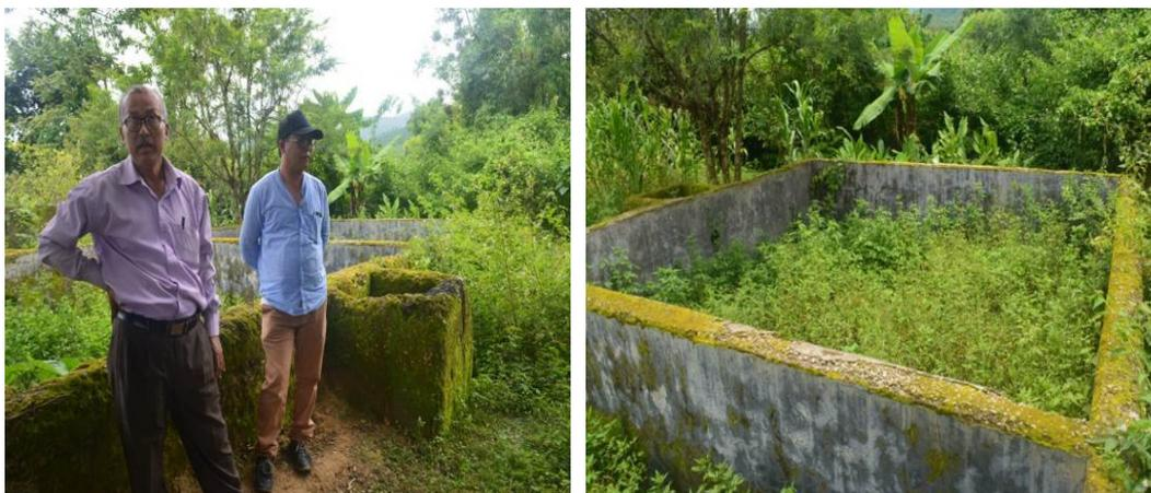
**Filter Media (left) and Settling tank (right) overgrown with grasses**
