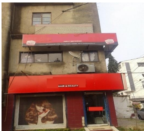
Figure 3.2: Encroachment in Kasba IEs by shops
