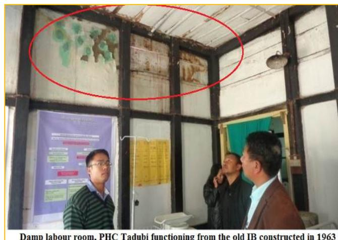
**Damp labour room, PHC Tadubi functioning from the old IB constructed in 1963**
