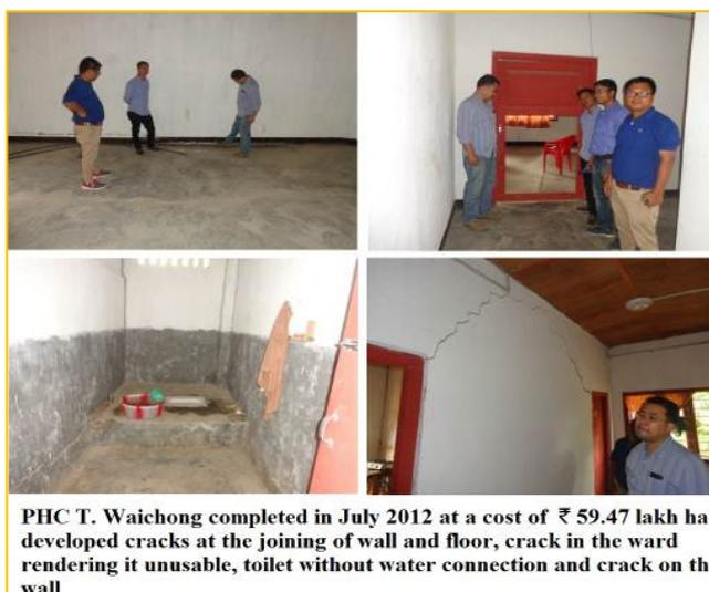
PHC T. Waichong completed in July 2012 at a cost of ₹ 59.47 lakh had developed cracks at the joining of wall and floor, crack in the ward rendering it unusable, toilet without water connection and crack on the wall
