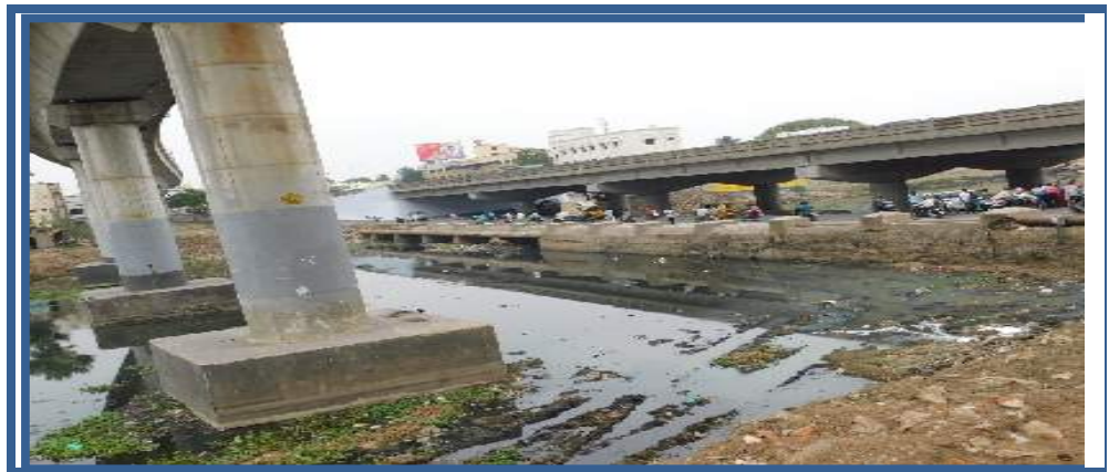
Exhibit 4.7: Metro Rail pile caps and old causeway
