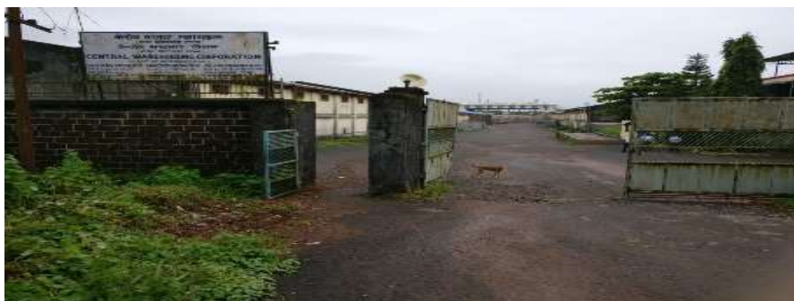
Photograph of single entry/exit gate at ICD Verna, Goa
