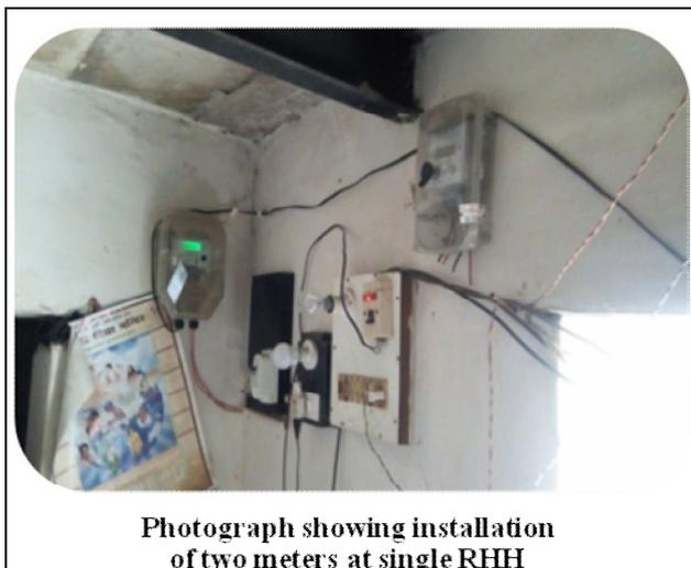
**Photograph showing installation of two meters at single RHH**
