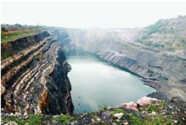
Fig. No. 3.8: Backfilling of Bengal Emta coal mines not done
