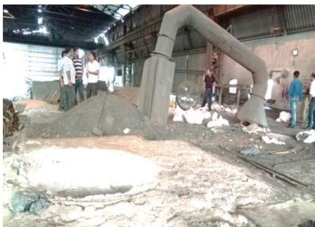
**Fig. No.3.4: Pollution control device in dilapidated condition in M/s. K B Sponge Iron Limited**
