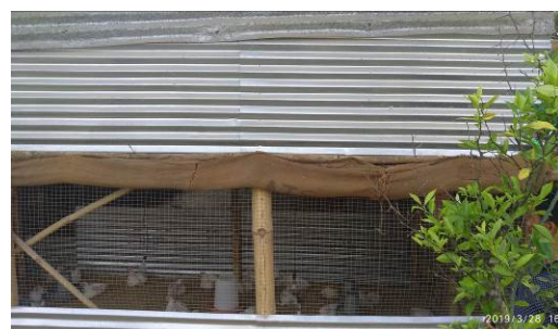
Structure constructed was being used as poultry house at the time of Joint Physical Verification. (28 March 2019)
