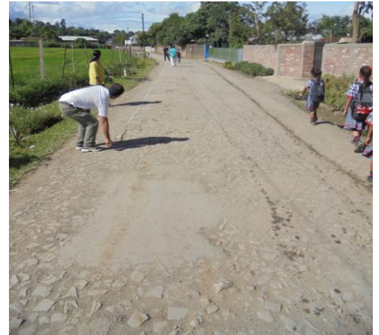
Improvement of Roads in and around Churachandpur District Hqrs (Worn out bituminous surface for a length of 200m at Marian street) (28 August 2018)
