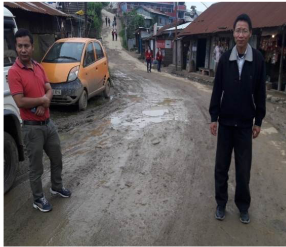
Improvement of Ukhrul District Hqrs road ( Damaged portion of Approach road to District Hospital) (12 July 2018)
