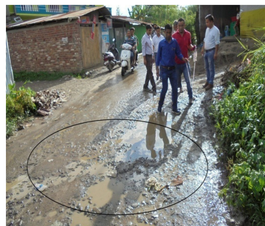
"Improvement of M.I. Bishnupur road and M.I. Bengoon" (Badly damaged portion of the work 'School Leirak, Ningthemcha Karong Road') (6 June 2018)
