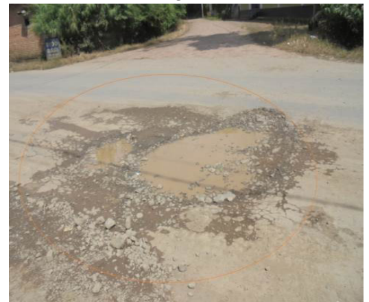
Improvement of Thoubal Charangpat Road via Nepra Company (Pothole at RD 7.8 km) (20 August 2018)
