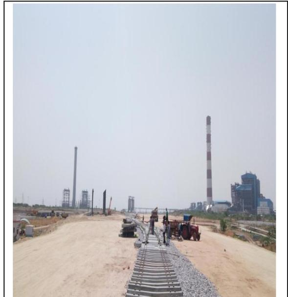
**Picture No. 2.1.2: Track laying in RSMY works**
