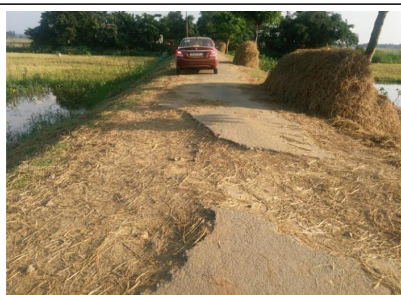
Picture showing broken road in the work 'Improvement i/c MBT of a road from AMPT road to Haribanga village via Bholarbita (0.300 Km) under RIDF-XX' which was completed during February 2017. Date of joint physical verification: 05.06.2018
