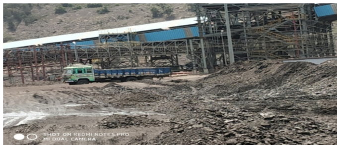
Pic. 05: Para No. 4.9.2: Idling of SILO at Lingaraj mine of MCL and resorting to road transportation.
