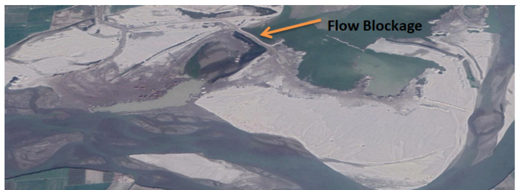
Damming of river flow in Gumthala North Block
