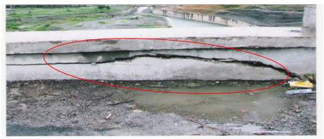
Crack developed in the retaining wall
