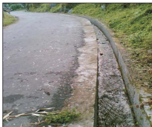
MIS at Tingvong serving as a roadside drain
