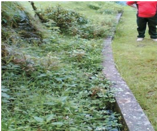
MIS at Ramathang in miserable condition due to non maintenance
