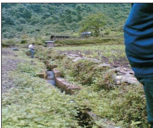
MIS at U/Khedum under Lachung serving only as a drain with fields on either side of it being above the level of the channel
