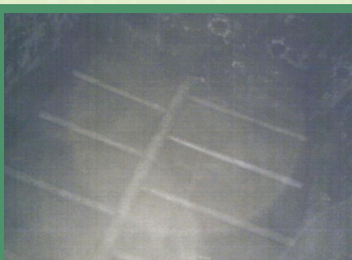
Rapid sand filter chamber without filter media
