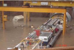
A length of 14.10 KM including lining was completed as of September 2012 out of 43.93 KM in Tunnel - I. The average boring rate targeted for both the TBMs put together was more than 1KM per month, while the achieved rate was only 210.45 meters due to power grid failure, non-availability of spares and frequent change of cutters of TBM.
