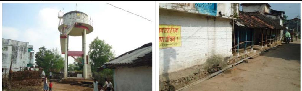
Over Head Tank constructed and GI pipeline can be seen laved at a cost of ₹ 6.50 lakh in October 2011 within village Ratanpur Girdhari, Raisen District from where household connection are provided. The PWSS is handed over to Mendki Panchayat of the village, having 115 individual household connections.
