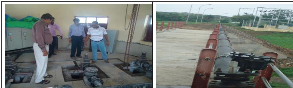
Intake well-cum-pump house and approach bridge to the intake well, installed pipe line, air valve and sluice valve installed at Village Velgipada, Sardarpur in Dhar district for covering 44 habitations in Badnawar/Sardarpur blocks of Dhar district for pumping raw water to the treatment plant, the work was completed in March 2013. After testing, water is being supplied since September 2013.
