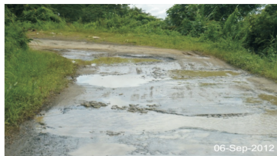
Stone filling and Water logging in Pot Holes in Lunglei – Tlabung Road (9.00 - 39.00 kmp)
