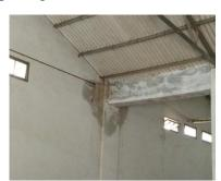
Picture 6: Leaky roof in Namakkal WH
