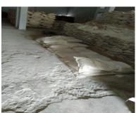
Picture 7: Damaged floor in Nagapattinam WH
