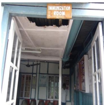
*Hole in ceiling of immunisation room Umsning CHC from where rain water leaks*
