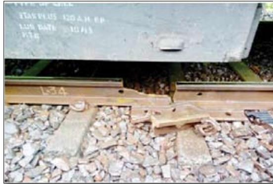
Figure 4: Rail fracture
