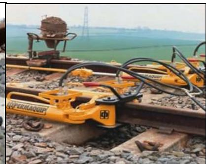
**Figure 10: Rail Creep Adjuster**
