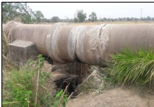
Bodhan ULB (Leakage from pipeline)
