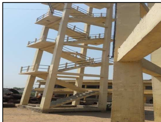
Non-provision of railings to stair case of 1 st and 2 nd flights of ELSR
