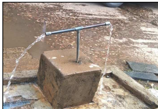
Manuguru ULB (Non-fixing of taps to the stand posts)
