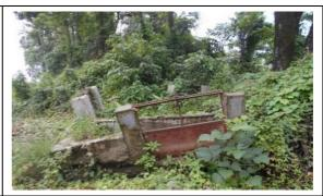
Damaged headwork at MIC at Inju Nallah (Sl. No. 8 of the table no. 2.2.7)
