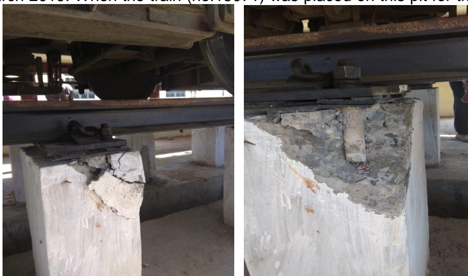
Figure 3.9 – Cracks/damage after placement of train in washing pit at Mau (18 March 2019)
