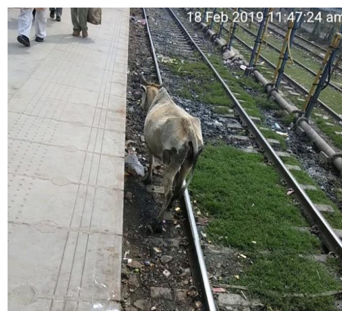
Figure 7.13 Incomplete fencing at Chheoki station leading to cattle on the tracks
